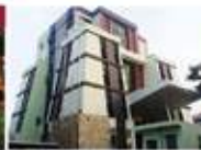
WATER BOARD (NWSD) REGIONAL OFFICE COMPLEX JAFFNA
